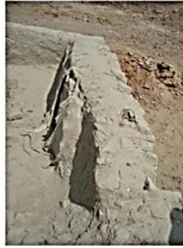
The successful use of the geo membrane, whose life is almost 100 years, this process is successfully used on the stopa area, where it has been, membrane and thin mud plaster is applied.
